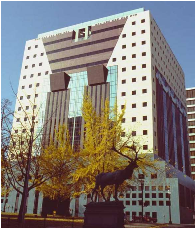
Public Services Building (Portland, 1982) Michael Graves
